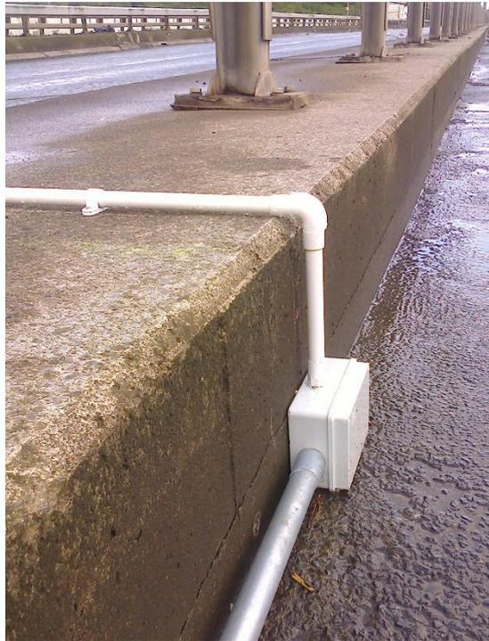
Figure 9 Conduit and IP Rated Joint Box
